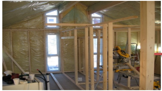
Building structure finished, Inside work on track
